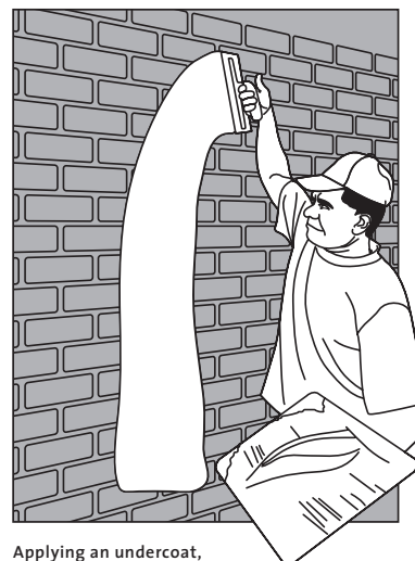
Applying an undercoat, one coat or multipurpose onto brickwork
